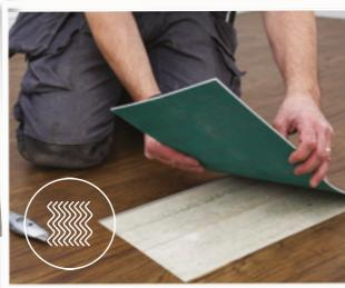
Our K-Wave+® friction grip backing allows the freedom to choose between pressure-sensitive or hard-set adhesives, providing flexible installation options to suit your individual needs.
